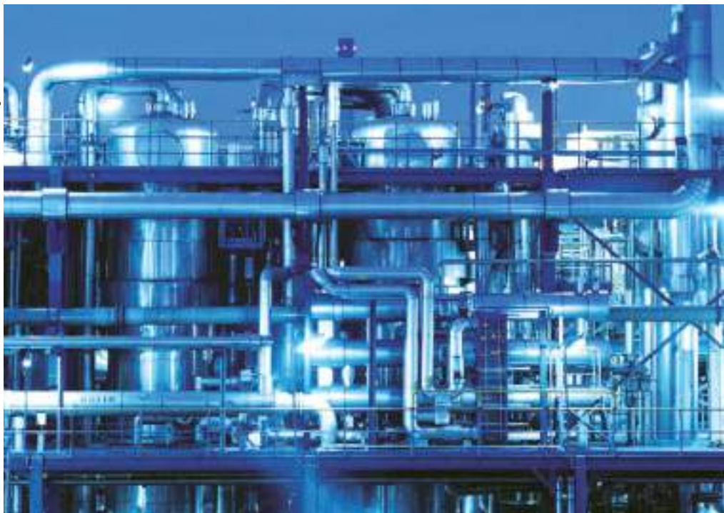
Pipe coatings play a critical role in preventing corrosion
