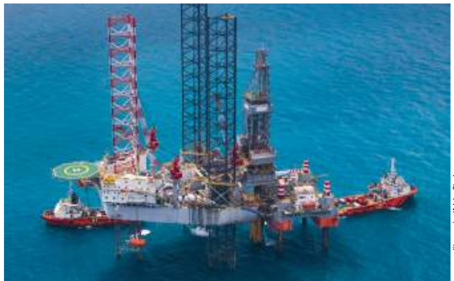
Increased production and discoveries are set to transform Egypt from a gas importer to exporter
