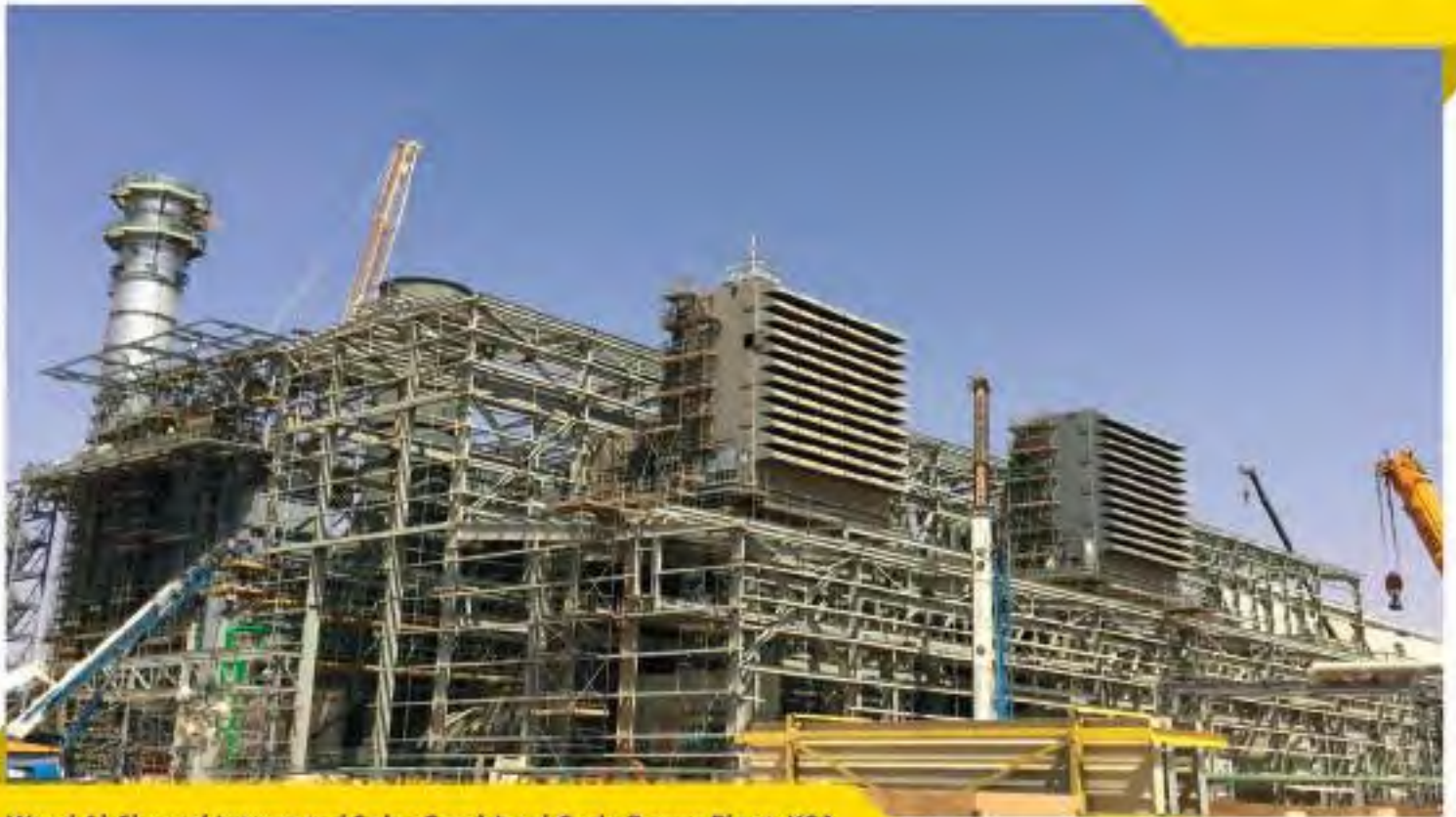
Waad Al-Shamal Integrated Solar Combined Cycle Power Plant, KSA
