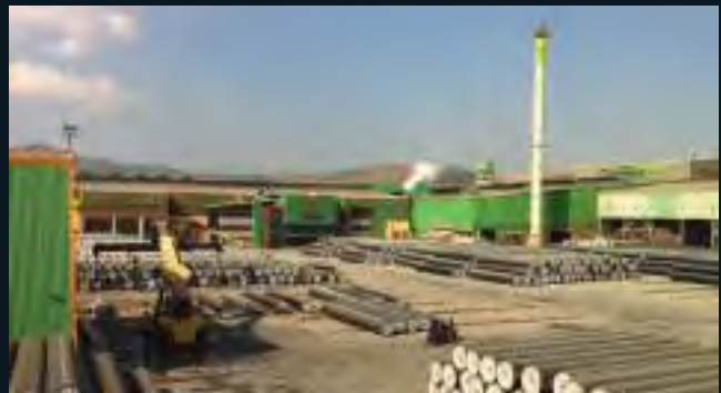
The group's facilities in Osmaniye
