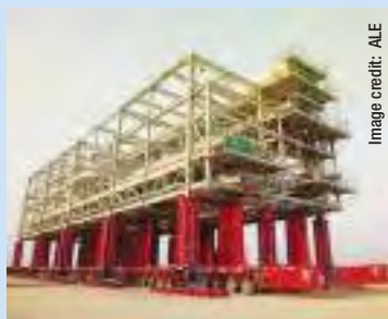
ALE's Mega Jack 300 jacking-up a 615t pipe rack module 5.9m using 15 bases with SPMTs underneath.
