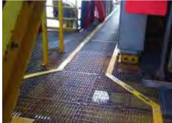
Safe Escape from Real Safety is anti-slip and mounted in the gratings of the rig
