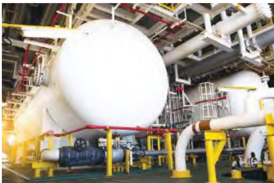
A production separator on an offshore oil and gas platform.
