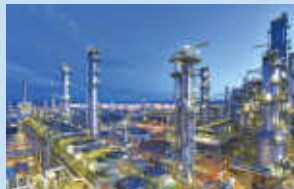
Reliable valves are essential in process control applications.
