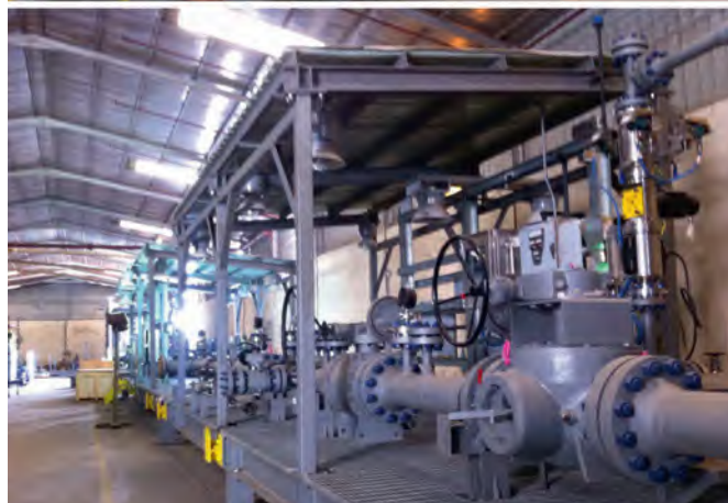
AES has state-of-the-art facilities in Saudi Arabia to build and commission water desalination plants and modular skids
