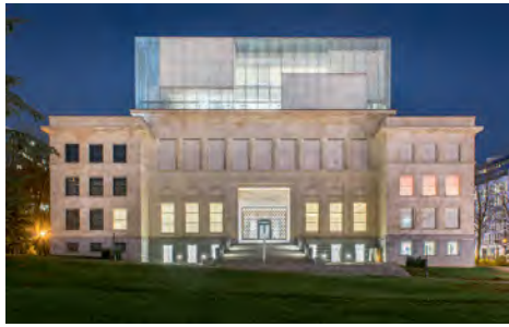
sedak's glass has been used in a number of iconic buildings
