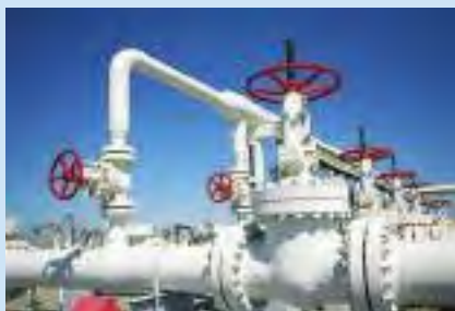
The LNG terminal will be set up in the Hidd Industrial Area. (Image source: INSAGO/Shutterstock)
