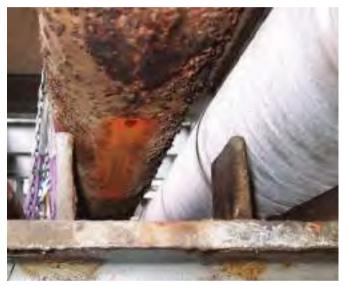
Fig. 1 - Evidence of pipe movement - early stage fretting/wear at the contact point
