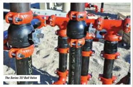
downstream applications, including the latest Victaulic Delta-Y Assembly, a combination of preassembled Victaulic cast grooved fittings, couplings and valves designed specifically for
