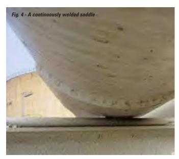
further corrosion, are leading some operators to provide direct access for inspection and remediation ("fabric maintenance") by support removal or line lifting. NDT techniques can be used to help manage the risks of pipework remediation, for example, by helping to determine whether the pipework can be safely re-supported, lifted, grit blasted and painted.
