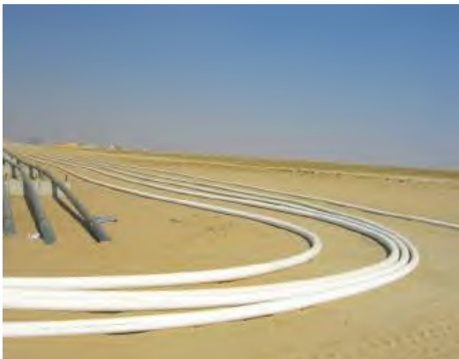
SoluForce FCP systems are flexible, meaning they can go up hills, down slopes, round corners and underwater with ease.
