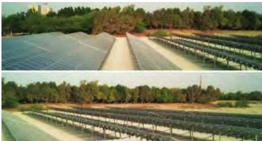
Bahrain has recently inaugurated a new solar energy pilot project (Photo: Bapco)
