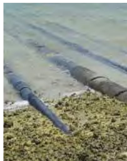
Pipeline in an intertidal zone
