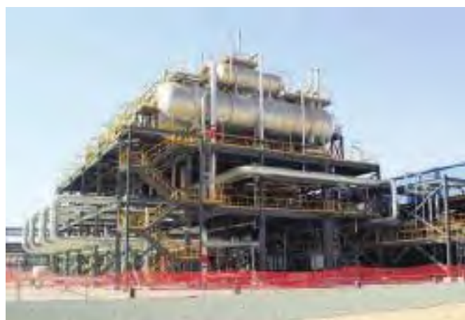
Wet gas fields are increasingly prominent in the Middle East
