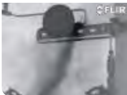
Methane gas leakage
