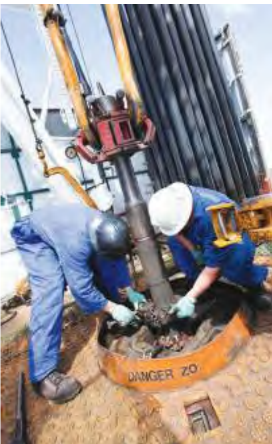
The majority of oil and gas workers are committed to the sector despite the downturn (Photo: DHL)
