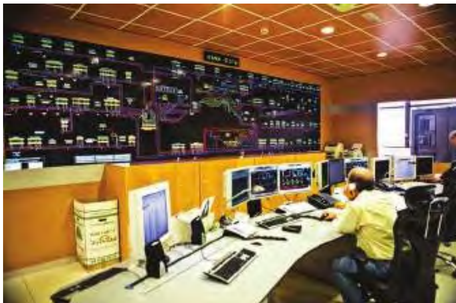
It is important to ensure controllers do not miss conditions and alarms that indicate a commodity release
