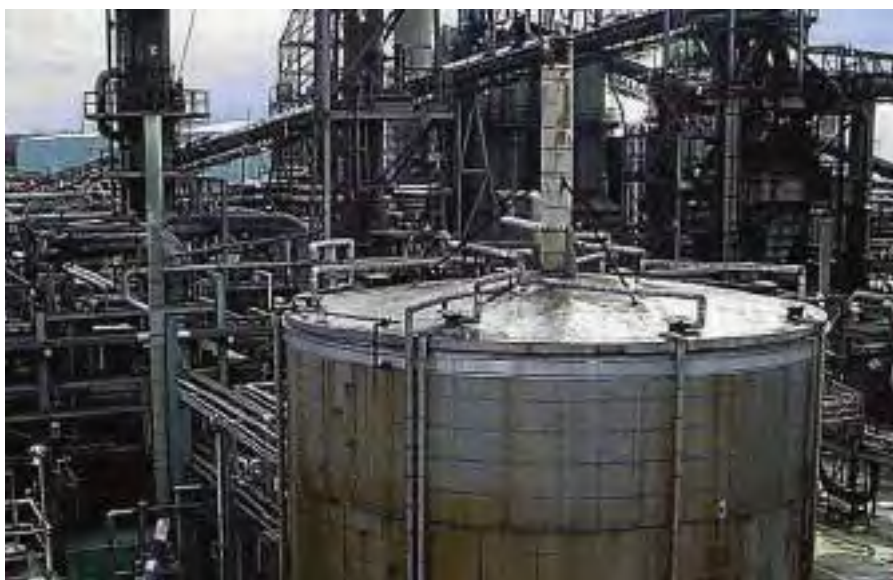
Sulfur storage tanks are plagued with corrosion issues
