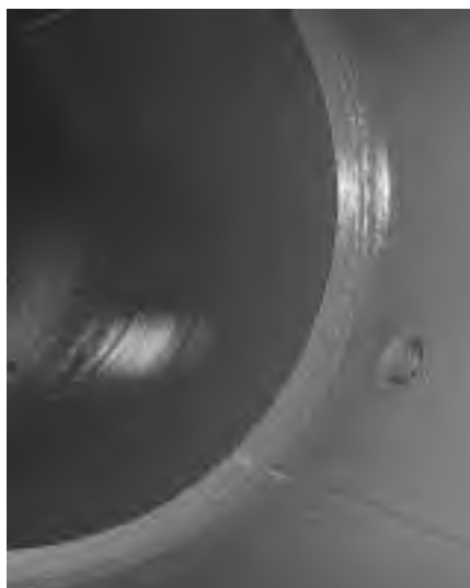
Complete application of Belzona spray-applied lining
