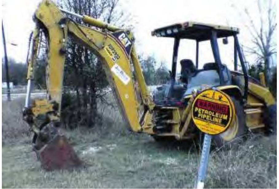
Many causes of commodity releases are associated with mechanical damage (Photo: Jeff Kramer)
