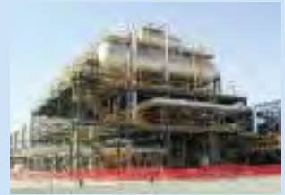
Abu Dhabi's Shah gas field contains sour gas
