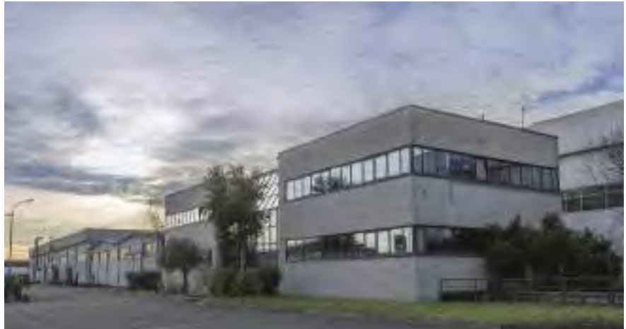
The Petrol Raccord plant
